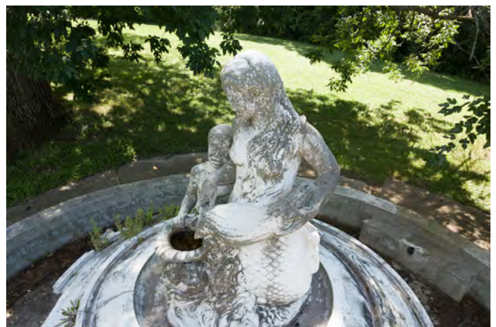
Figure 13: View of mermaid and cornucopia - note the apparent loss of detail from organic buildup
