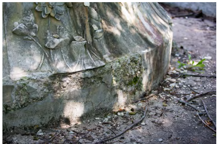
Figure 31: Stone to concrete transition
