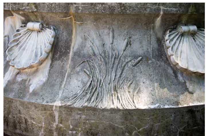
Figure 34: Relatively intact stone to concrete transition
