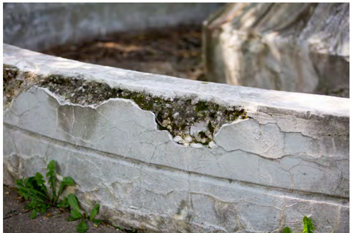
Figure 24: Coarse ring aggregate concrete at lower perimeter
